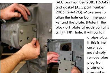
208512-A42G). Make sure to align the hole on both the gasket and the plate. (Note: If the block off plate already contains a 1/4"NPT hole, it will contain a pipe plug. If this is the
